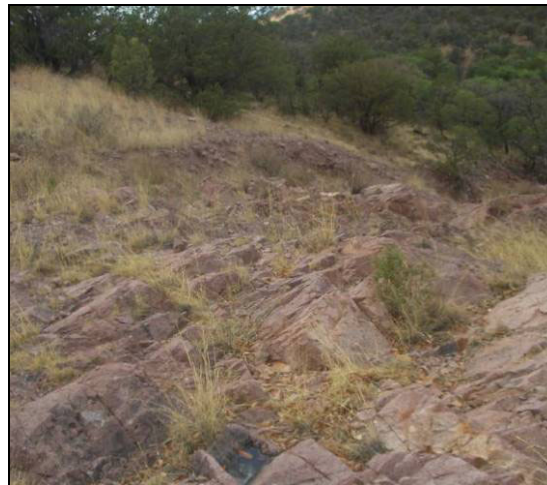
Figure 7.4 Photograph of the back of spillway. The lack of erosion and sedimentation indicates infrequent use of spillway.
