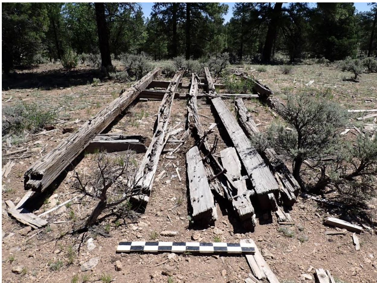
Figure 12: Overview of Locus I building foundation, facing north. Photo by Damon Marcinko.
