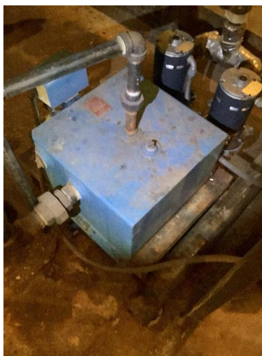
Fig 7: Condensate Tank/Pumps
