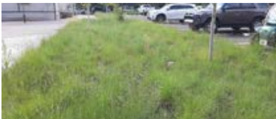
Detention and snow storage basin vegetated with blue grama meadow
