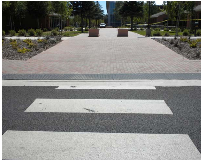
Photo 2: Truncated dome surface at walkway
