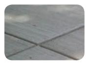
Concrete Paving Broom Finish
