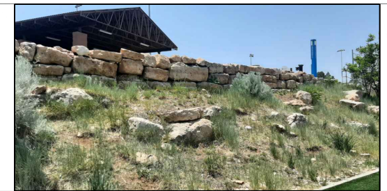
DRYSTACK LIMESTONE RETAINING WALL
