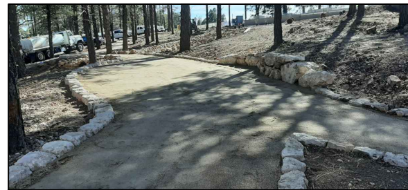
CRUSHER FINES WITH LIMESTONE EDGE BORDER
