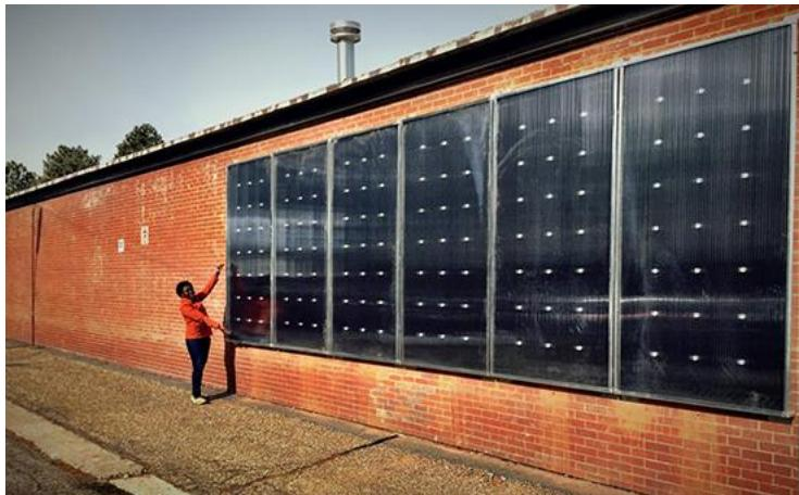
Property surplus is outfitted with six solar powered hot air heaters. This technology supplements the traditional natural gas system within the building. This project lowers our CO2 emissions by 3 tons a year and tests a renewable heating option for the campus.
