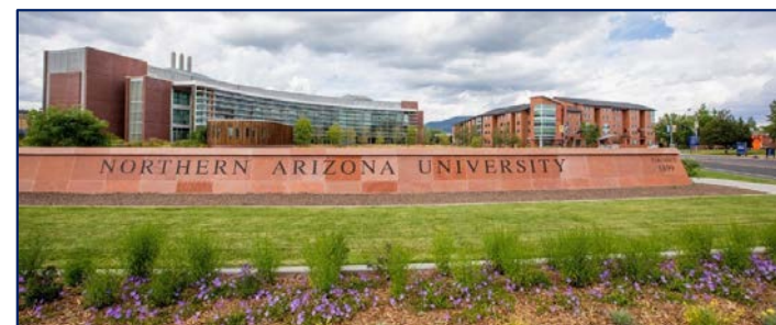
Applied Research and Development
