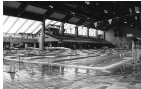
Douglas J. Wall Aquatic Center
