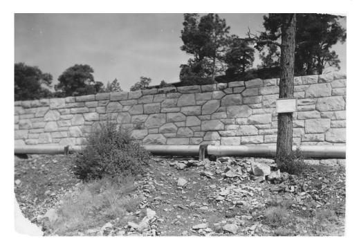
Figure 54: New retaining wall constructed by CCC where old steam lines crossed Hermit Rim Road, 1935, GRCA 7820.
