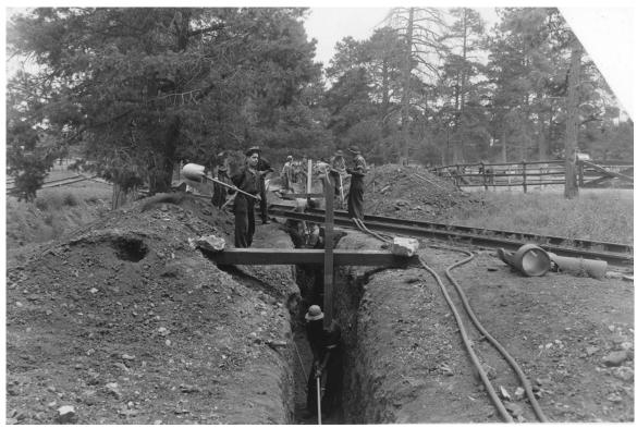
Figure 28: Sewer trenching under railroad tracks, 1935, GRCA 253.
