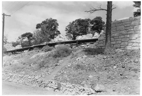
Figure 56: Steam pipes through wall leading to Bright Angel Lodge, 1935, GRCA 6172.
