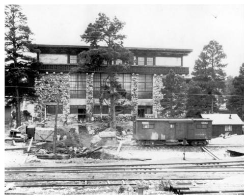
Figure 44: Powerhouse construction with open pipe trench, ca. 1926, GRCA 13115.
