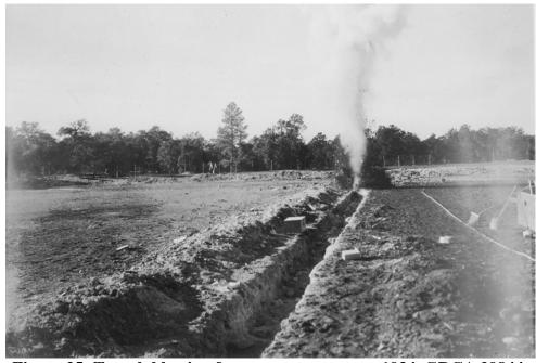
Figure 25: Trench blasting for new water system, 1934, GRCA 29844.
