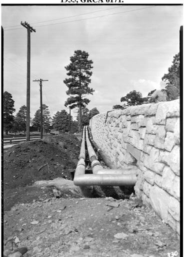
Figure 53: CCC extension of steam and ammonia lines to pipe chase, 1935, GRCA 330.
