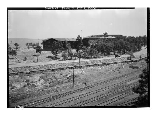
Figure 55: Steam/ammonia/conduit to El Tovar after realignment, also note electrical lines and aboveground water pipe, GRCA 653.
