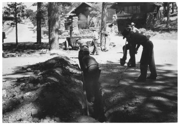
Figure 15: CCC crew constructing water pipe trench to Building No. 1, ca. 1935, GRCA 6610.
