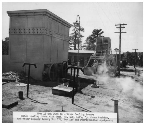
Figure 63: Both water cooling towers, 1953, GRCA 1953\_report\_14-15.
