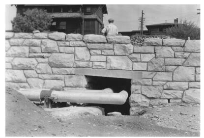
Figure 52: CCC-constructed pipe chase for El Tovar carrying steam and ammonia lines, 1935, GRCA 6171.
