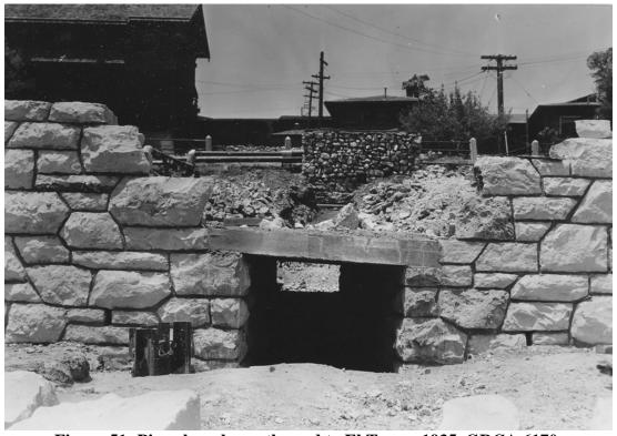
Figure 51: Pipe chase beneath road to El Tovar, 1935, GRCA 6170.
