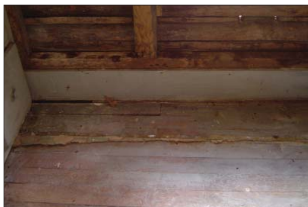
Fig. 49: Northeast corner of Room Two showing linoleum flooring over wood, 2006.
