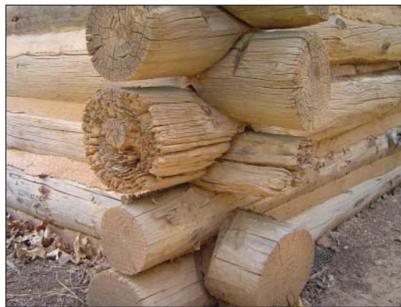
Fig. 38: Decayed crowns at northeast corner, 2006.
