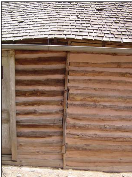
Fig. 32: Connection between original cabin and second addition does not provide adequate structural support, 2006.
