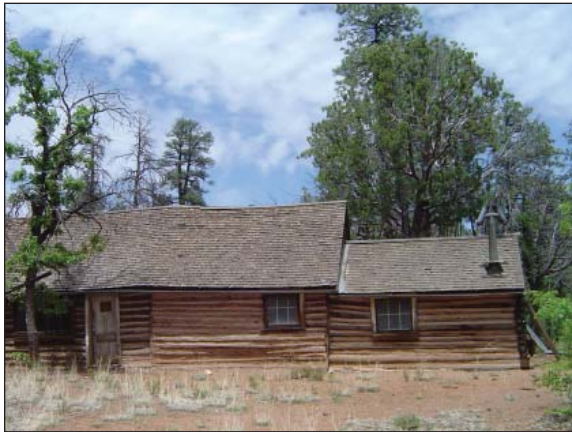
Fig. 30: South elevation showing ridge in roof between original cabin and second addition, 2006.
