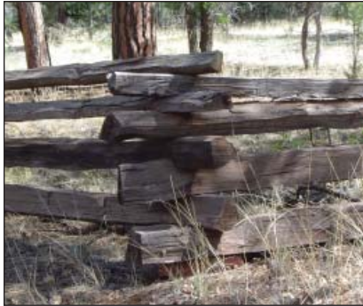
Fig. 6: Typical connection along Boundary Fence, 2006.
