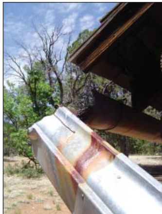
Fig. 41: Blocked gutter at southeast corner, 2006.
