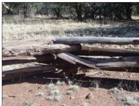
Fig. 13: Failure and collapse at junction, 2006.
