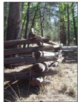
Fig. 11: Combination of full and split logs, 2006.
