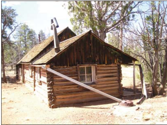
Fig. 39: East elevation showing drainage toward building and displaced gutter, 2006.
