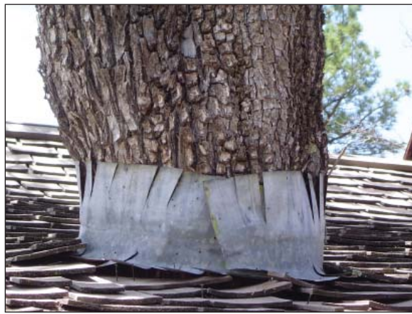
Fig. 42: Flashing around tree at kitchen roof does not provide water-proof seal, 2006.
