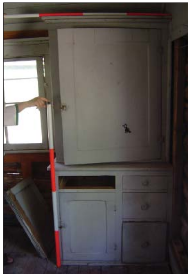
Fig. 51: Built-in storage showing missing drawer and damage to west side, 2006.
