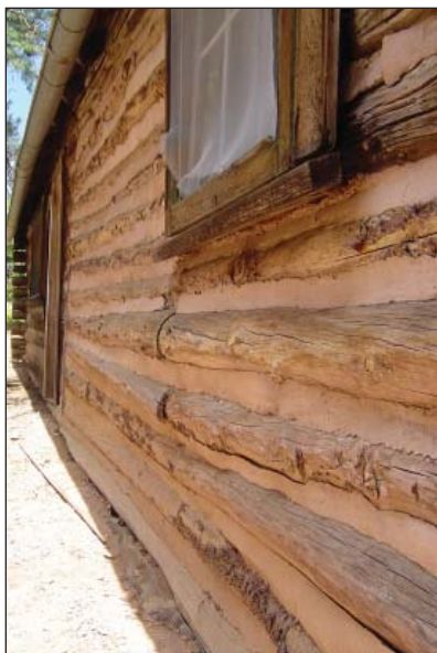
Fig. 34: Bowed wall under window on original cabin where historic chimney once existed, 2006.
