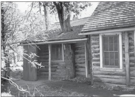
Fig. 12: Ranger Cabin with corrugated sheet metal at kitchen porch corner and exterior bracing, April 1988 (WACA 2373)
