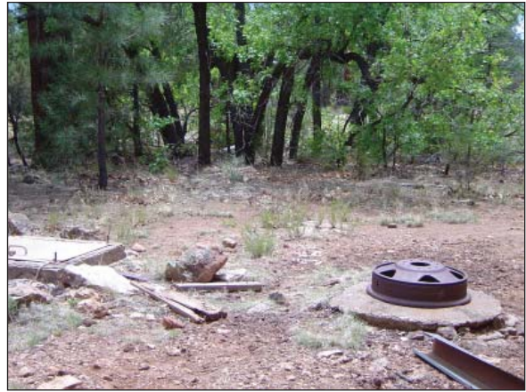
Fig. 40: Cement-capped cistern with locked hatch at left and water catchment at right, 2006.
