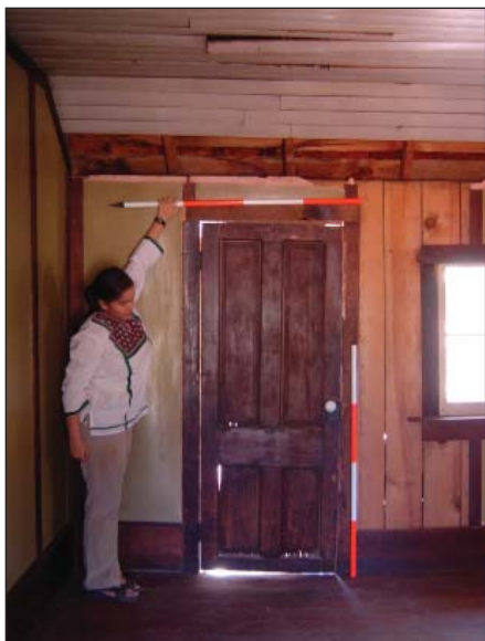
Fig. 53: North wall of Room Three showing ceiling damage, missing wallboard, and dark stained trim, 2006.
