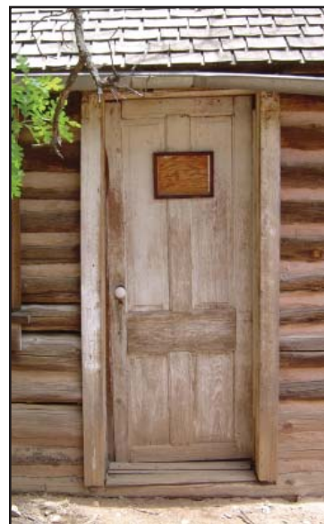
Fig. 36: Door askew on the south elevation of the second addition, 2006.
