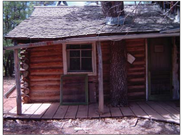
Fig. 31: Kitchen addition on north elevation showing improper roof slope, 2006.
