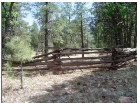
Fig. 9: Section of Boundary Fence parallel to road and five logs high, 2006.
