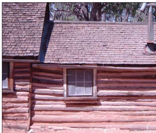
Fig. 37: South elevation of kitchen addition showing improperly tied logs angled toward window, 2006.
