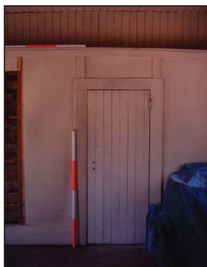
Fig. 46: East wall of Room One showing recess and shelf above original exterior wall, and irregular height beadboard door, 2006.
