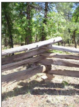
Fig. 15: Bottom logs rests upon two stones, 2006.
