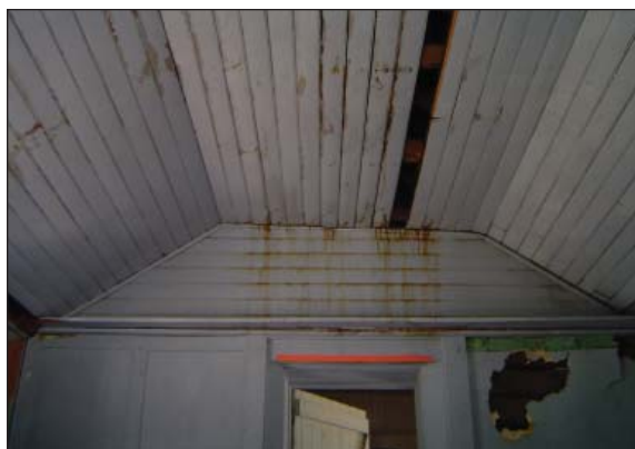
Fig. 48: West wall and ceiling of Room Two showing ceiling and wall damage, including presence of unidentified sticky substance, 2006.
