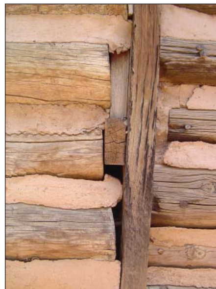
Fig. 33: Detail of connection between original cabin and second addition showing logs attached to a vertical wood post, 2006.
