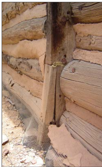
Fig. 35: Cracked member at hog-trough corner between original cabin and kitchen addition provides inadequate structural stability, 2006.
