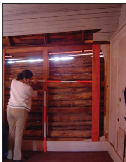
Fig. 45: South wall of Room One showing ceiling damage, missing wallboard, and exposure to exterior, 2006.
