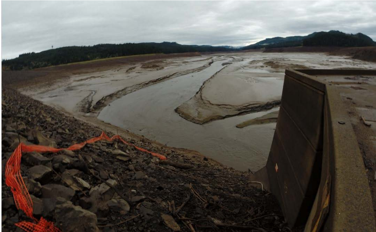
Figure 2. Annual fall deep drawn down to support fish passage at Fall Creek Reservoir
