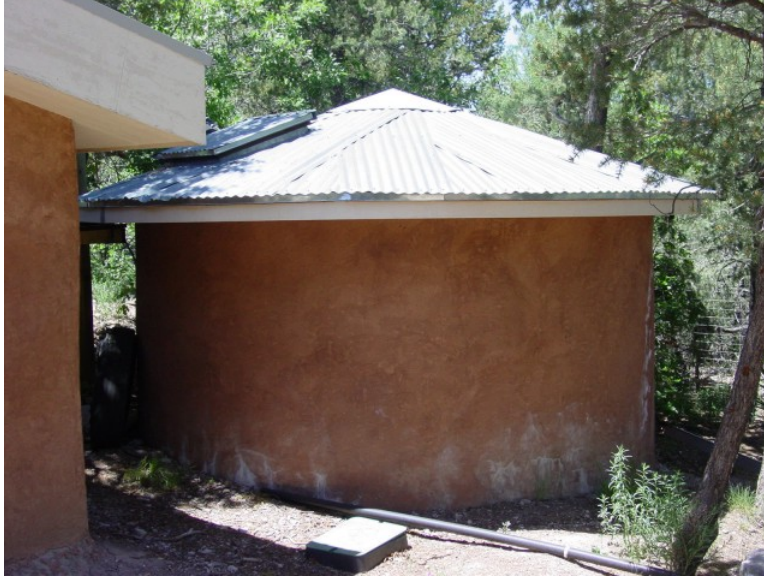
Fig. 2. Ferro-cement Rainwater Cistern ( http://www.soilutions.net ).
