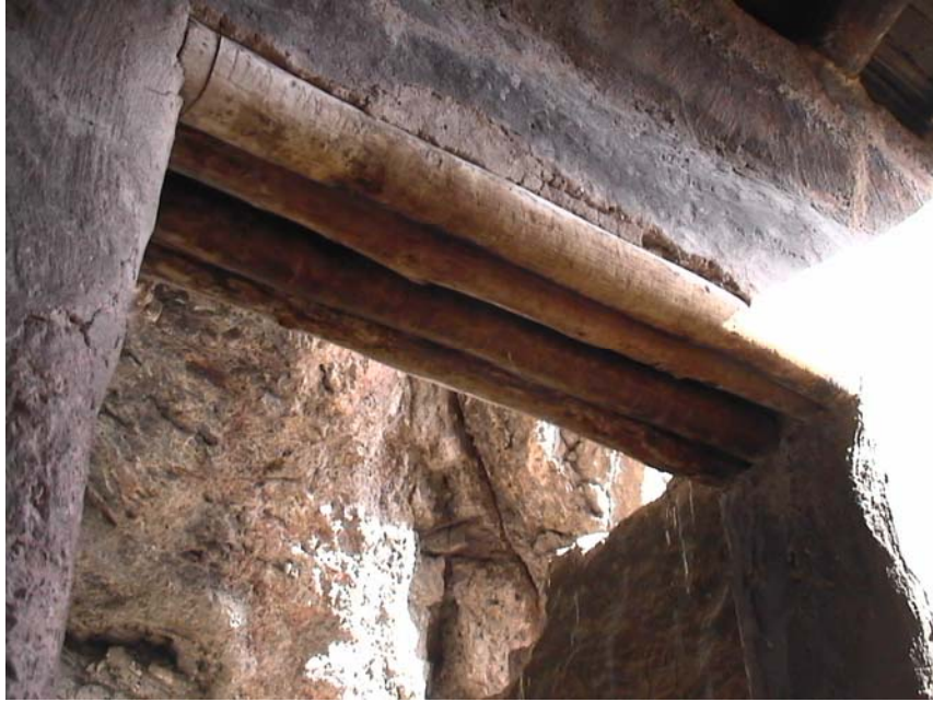
Figure 8. Replaced pole lintels at Lower Cliff Dwelling, north doorway, room 9. Replaced by Gordon Vivian, 1952.
