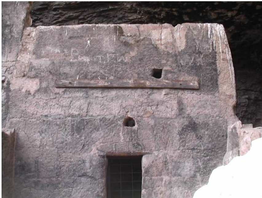
Figure 9. 2x6 used to stabilize room 15 east wall, Lower Cliff Dwelling. Installed by Roland Richert, 1957.
