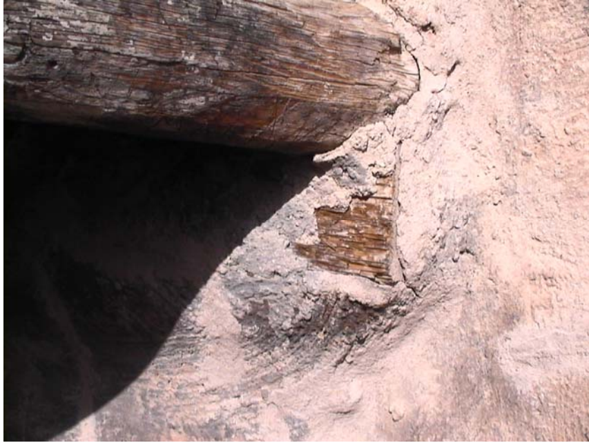
Figure 6. Exposed corner of stabilized 2x4 above doorway,, Lower Cliff Dwelling, Room 9, north wall. Installed by Gordon Vivian, 1952.
