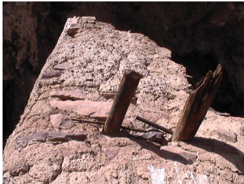
Figure 7. Replaced dowel pin in exposed viga, Lower Cliff Dwelling, room 1, north wall. Replaced by Faye Morrison, 1992.
