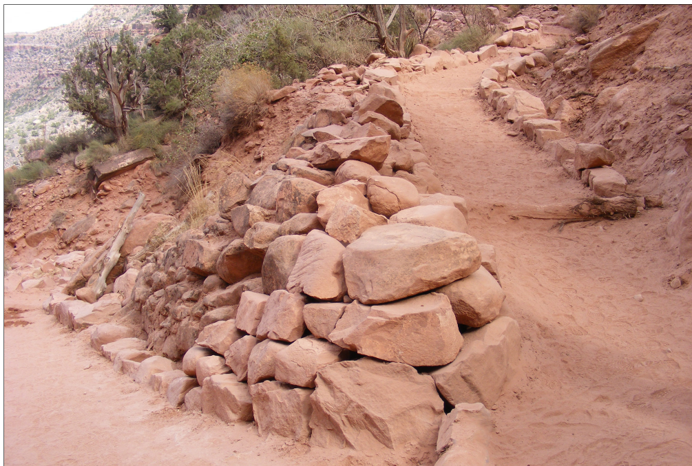
Photograph 10. Switchback with dry-stacked stone infill, looking north, 2009. Source: Logan Simpson Design (LSD).
