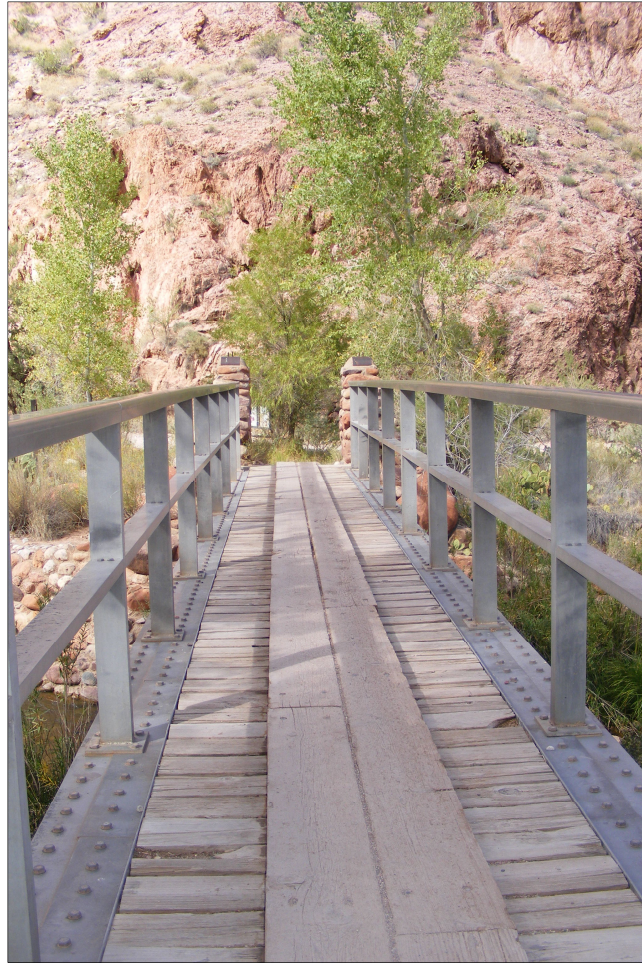
Photograph 8. Bridge crossing at Bright Angel Creek, showing steel rails and wood plank decking, looking northwest, 2009. Source: Logan Simpson Design (LSD).
