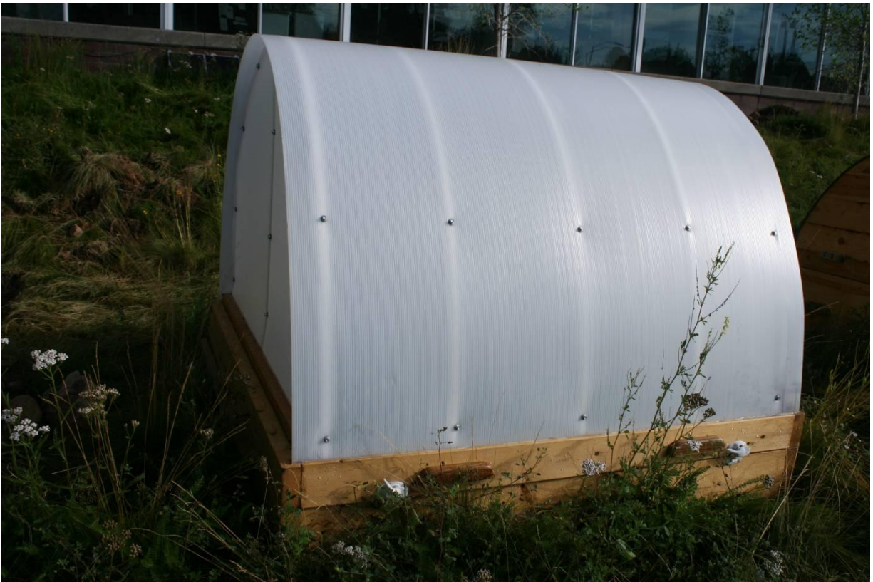
Figure 47: Structure #10 - Hooped Pod with Solexx
