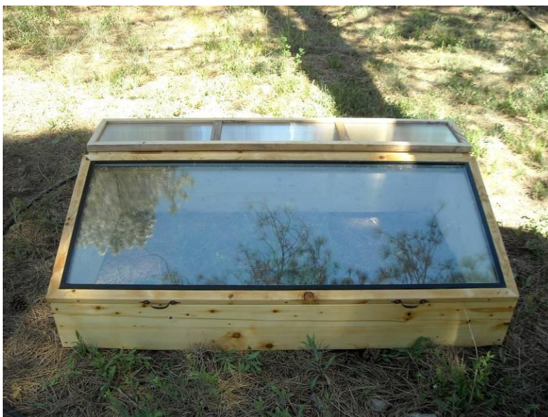
Figure 39: Structure #2 – Cold Frame with Foam Board Insulated Walls
