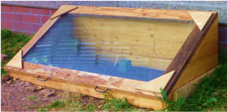
Figure 42: Structure #5 – Cold Frame with 27° Angled Lid
