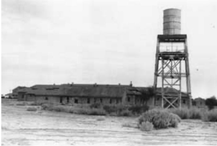
Sixty-foot water tower at Leupp Boarding School. Museum of Northern Arizona photo archives.
