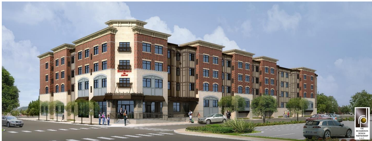
Example of a large-scale commercial block building
