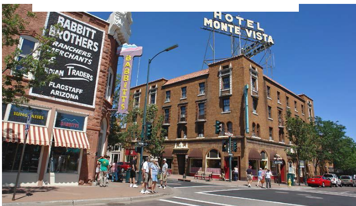
Example of a medium-scale commercial block building
