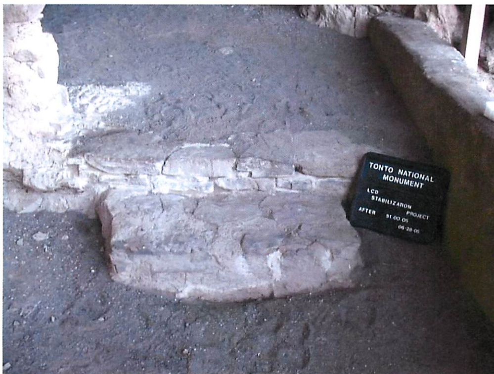
Figure 14. After photo of NPS construction 51.00.05NPS.
