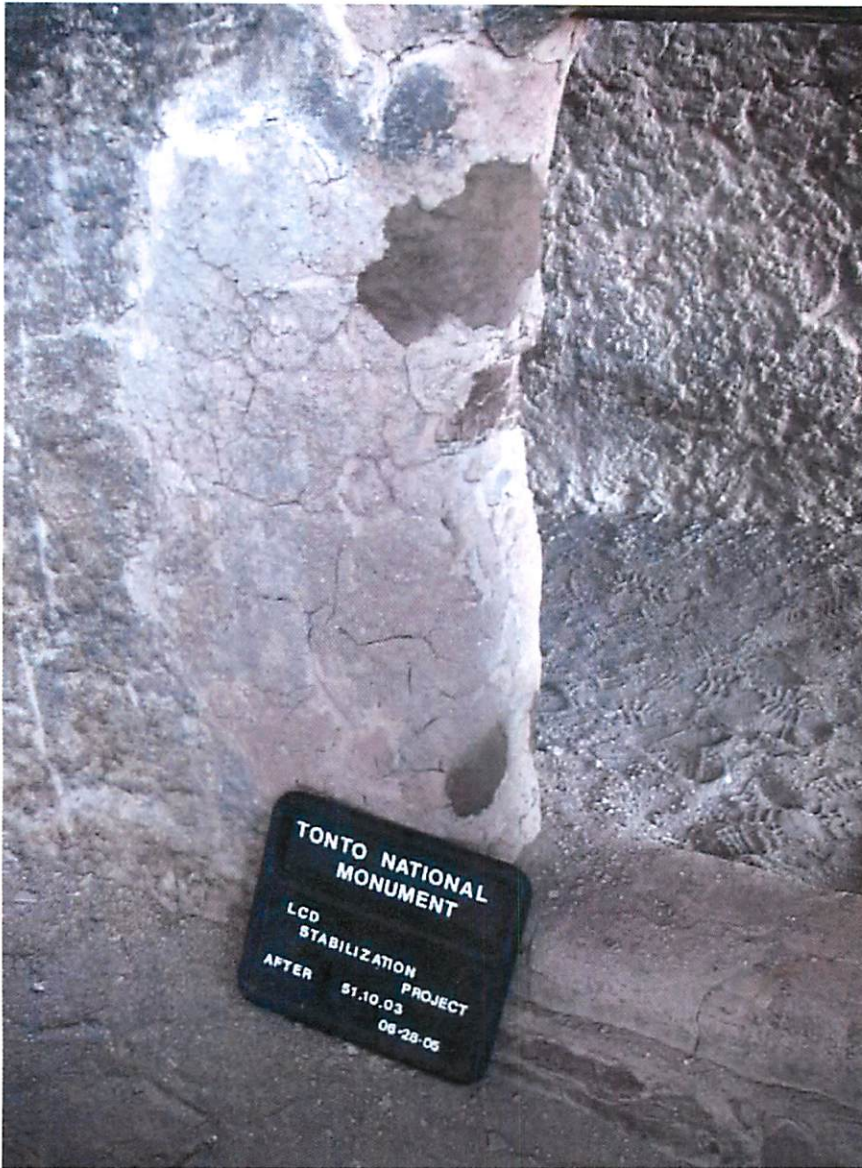
Figure 8. After photo of wall 51.10.03, detail area of doorway between Rooms 9 and 10.
