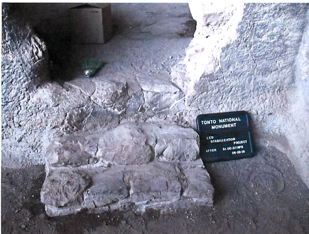
Figure 18. After photo of NPS construction 51.00.07NPS.
