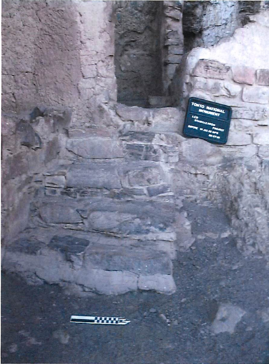
Figure 11. Before photo of NPS construction 51.00.02NPS.
