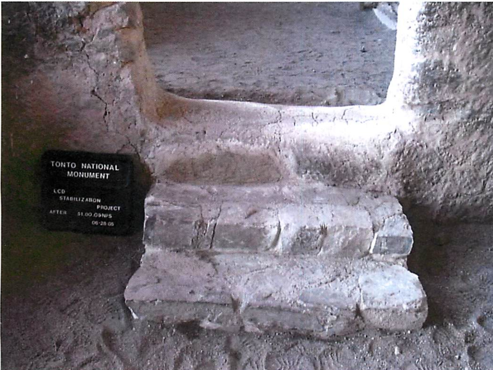
Figure 21. After photo of NPS construction 51.00.09NPS.
