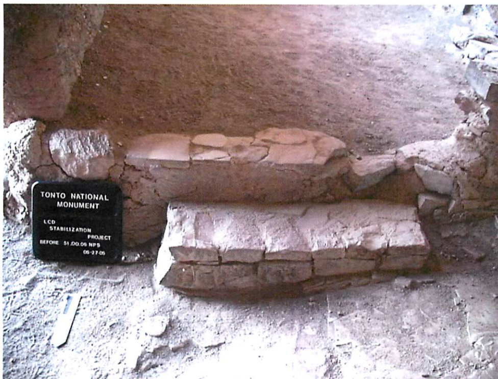
Figure 15. Before photo of NPS construction 51.00.06NPS.
