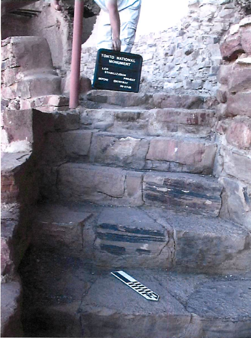
Figure 24. Before photo of NPS construction entryway steps.
