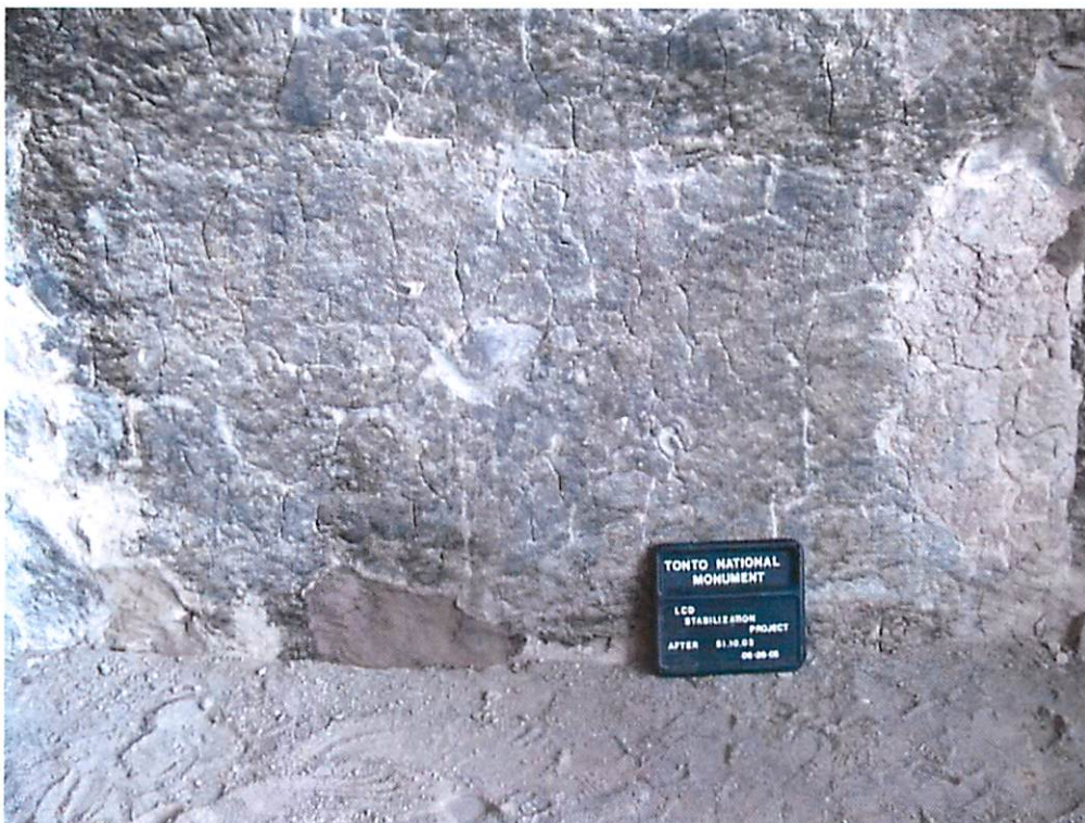
Figure 7. After photo of wall 51.10.03.
